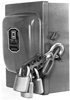
Fig 9.2—If the switch box feeding power to your shack is equipped with a lock-out hole, use it. With a lock through the hole on the box, the power cannot be accidentally turned back on. (Photos courtesy of American ED-CO, at top, and Osborn Mfg Corp, at bottom)
